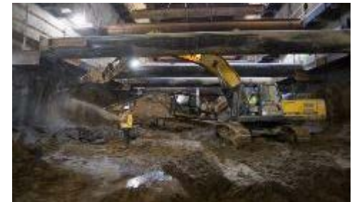
Union Square Station Construction
