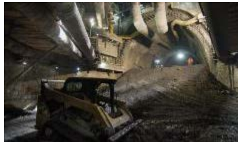
Chinatown Station Construction
