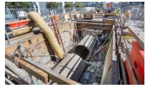
Surface Work ~ Sewer Replacement @ 4 th Street
