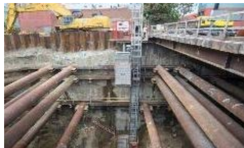
Moscone Station Construction
